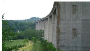
the quality of the concrete cover and the content of the chlorides around the reinforcement will cause similar corrosive circumstances. These circumstances will cause local corrosion cells. These locations are anodic. Other locations of the reinforcement, where the circumstances are relatively less corrosive and aggressive, remain passivated (passive oxide-layer). These locations are cathodic.
