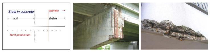
European standard ISO 12696: "*Cathodic Protection of steel in concrete*" details the principles of CP and its application to steel in concrete. The purpose of cathodic protection of steel reinforced concrete is to suppress the corrosion process of steel in concrete by use of an applied current.
